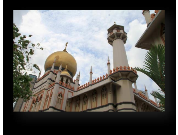
Masjid Sultan, Sultan's Mosque
